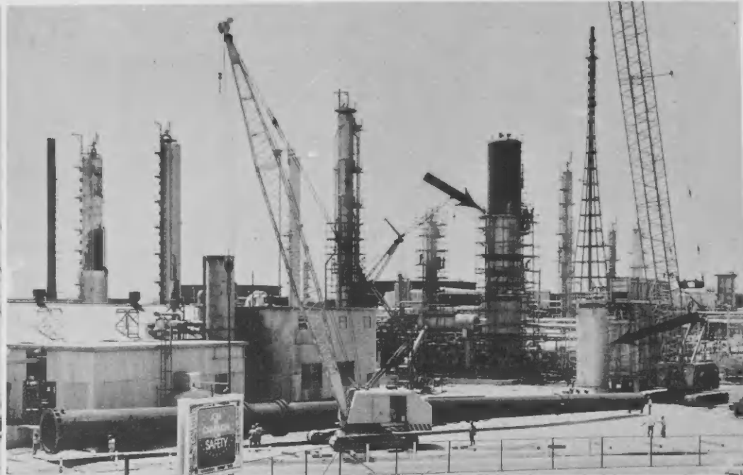
At left, the old section of the 83-ft high splitter tower before removal. At right, preparations are made to take down the furnace stack.
